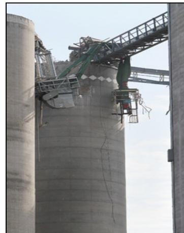
Damage to a grain elevator from a combustible dust explosion
